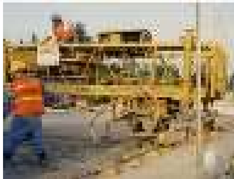
Gambar 27-l. Traversing roller tube paver
