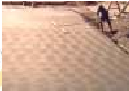
Gambar 28- ee. Straightedging behind a longitudinal float
