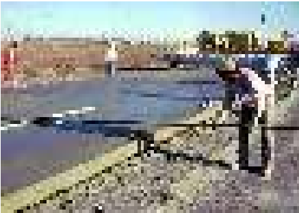
Gambar 28- dd. Pushing the straightedge – keeping the handle low
