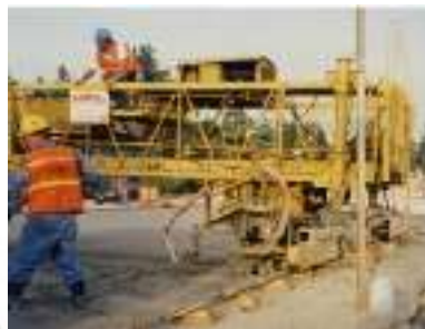
Gambar 15 Transversing roller tube paver
