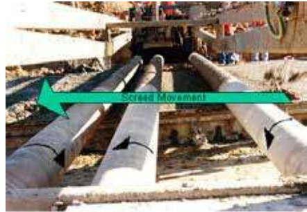
Gambar 14 A Clary or Roller Screed
