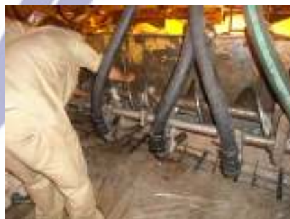
Gambar 79 Instrumen vibrator
