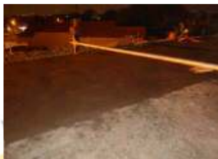
Gambar 77 Lean concrete tebal 10 cm
