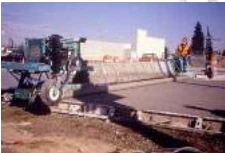
Gambar 11 Self-propelled roller screed
