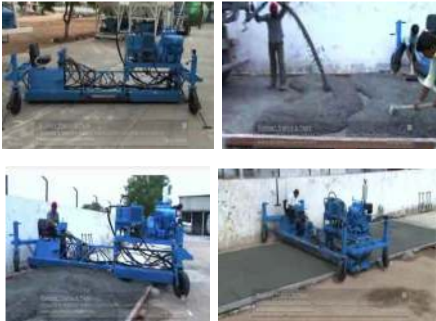
Gambar 2 Apollo Fixed Form Concrete Paver di India (Sumber: http://www.youtube.com/watch?v=ms0mcTxMAHo )
