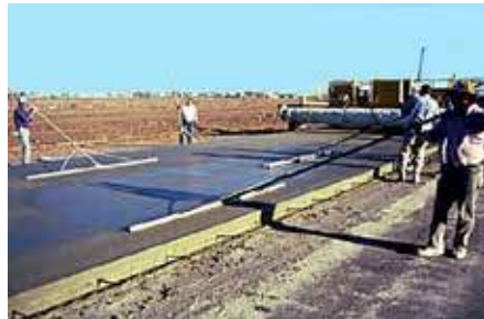
Gambar 64 Pulling the straightedge – keeping the handle high
