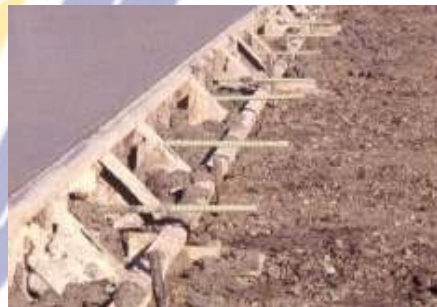
Gambar 12 Tie bar dipasang manual
