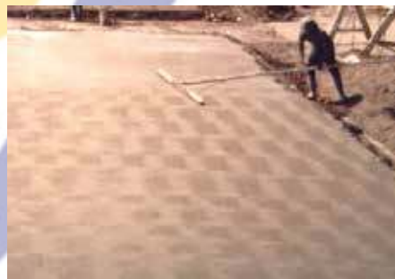
Gambar 66 Straightedging behind a longitudinal float
