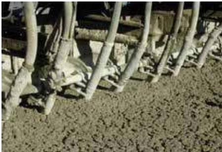
Gambar 52 Vibrator terbenam ( Immersion Vibrators ).
