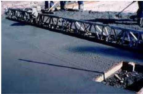
Gambar 13 Vibrating screed
