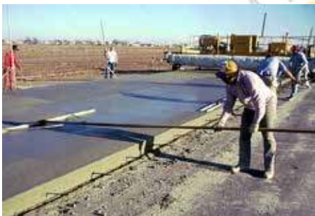
Gambar 65 Pushing the straightedge – keeping the handle low
