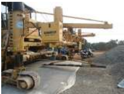
Gambar 77 Lean concrete tebal 10 cm
