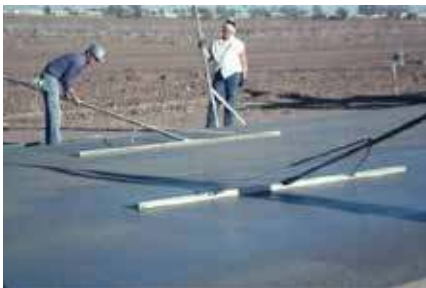
Gambar 63 Straightedge Finishing
