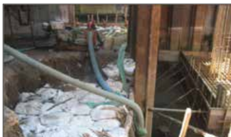
Gambar 4.25 Proses Dewatering
