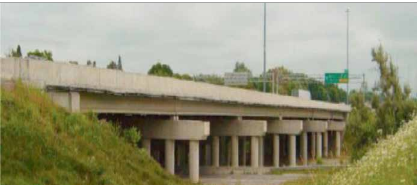
Gambar 2.21 Jembatan Duffin creek deck
