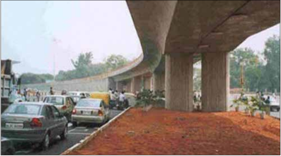
Gambar 1.1 Jembatan Integral Flyover Kalkaji
