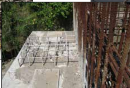
Gambar 4.33 Pengecoran abutment
