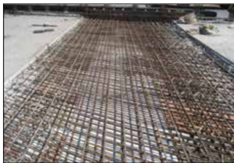
Gambar 4.19 Pengecoran deck slab
