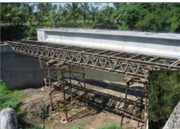
Gambar 4.32 Launching Girder
