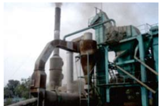
Gambar 3.5 Elevator Panas ( Hot Elevator )
