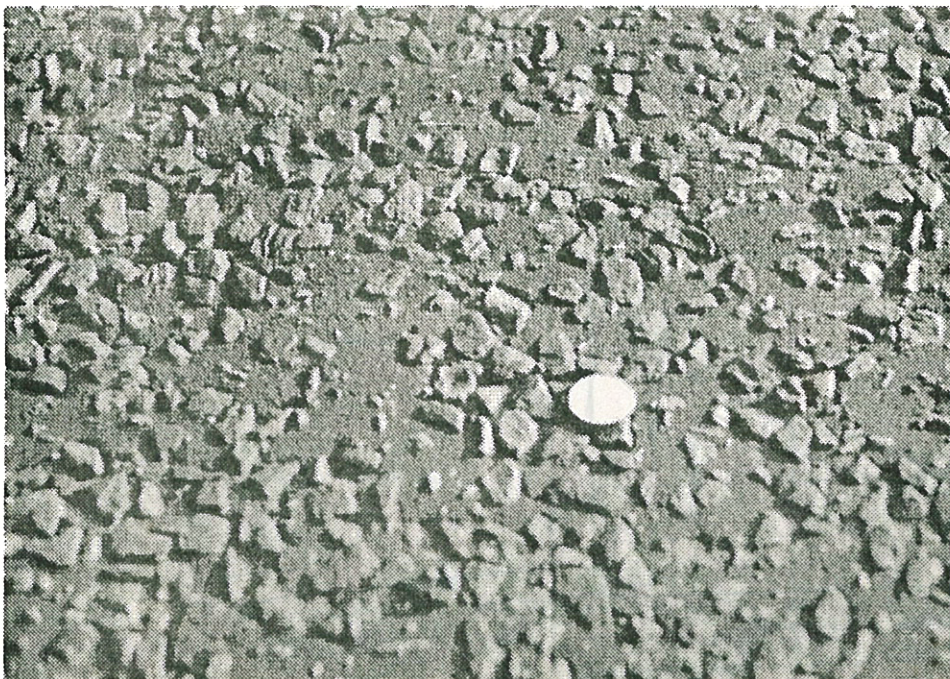
Fig. 4. Detail HRA type wearing course using lightly chipped( 20 m )
