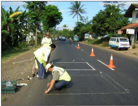
Gambar 3. Sensor weigh in motion system
