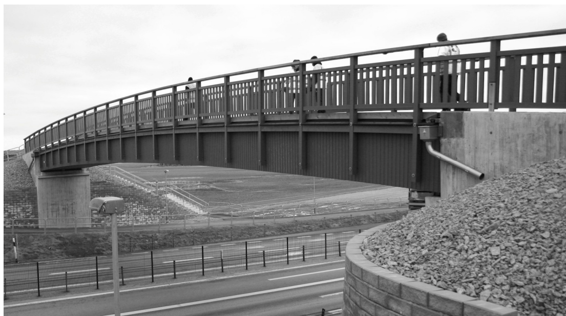
Figure 5.4 Stolpen bridge, spanning over the motorway E18, between Oslo and Stockholm. Photo: Carl Westerlund
