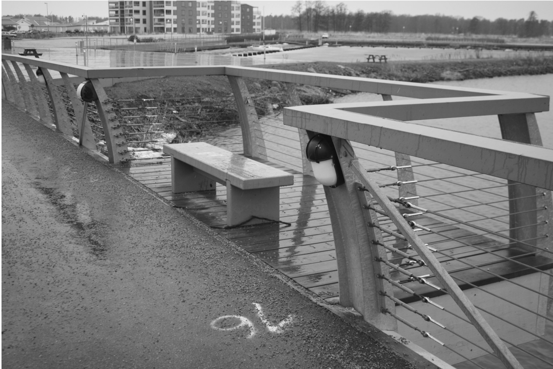
Figure 5.9 One of the balconies on the multi-span bridge.
