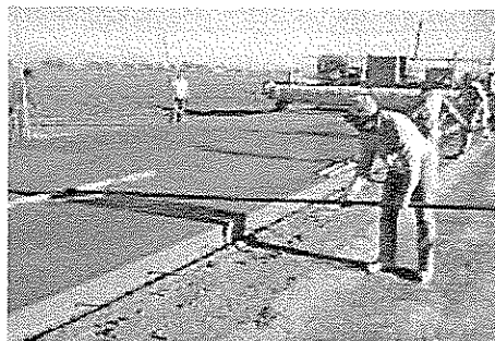
Gambar 59 Pushing the straightedge – keeping the handle low
