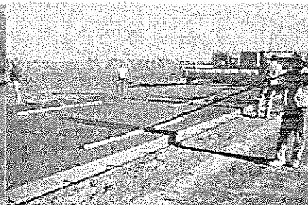
Gambar 58 Pulling the straightedge – keeping the handle high
