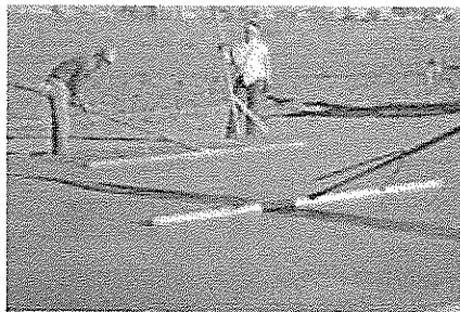
Gambar 57 Straightedge Finishing
