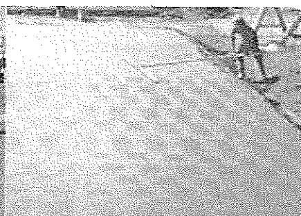
Gambar 60 Straight edging behind a longitudinal float
