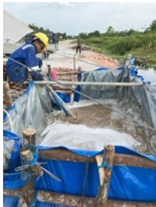
Drilling Fluid Storage for Hybrid Drilling Method
