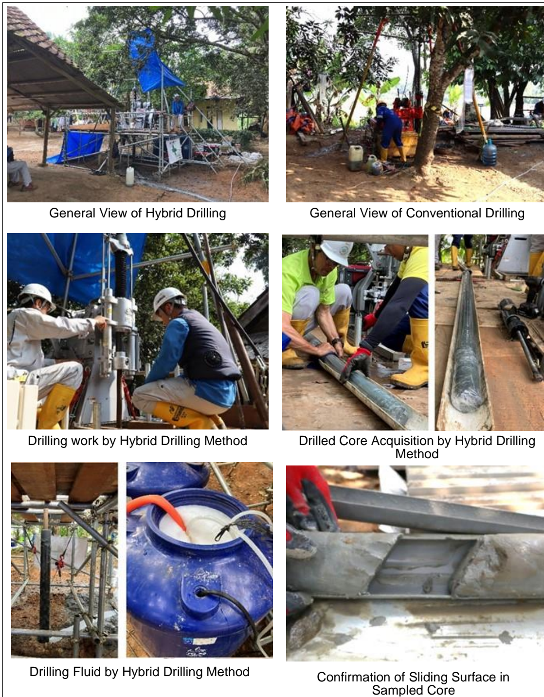
Figure 2-2. Photographs of drilling work at Serang-Panimbang Toll Road Site
