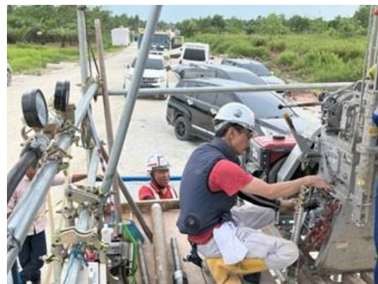
Drilling Work by Hybrid Drilling Method
