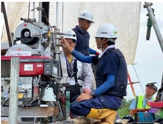
Drilling Work by Hybrid Drilling Method
