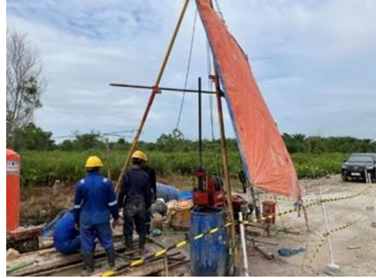
General View of Conventional Drilling
