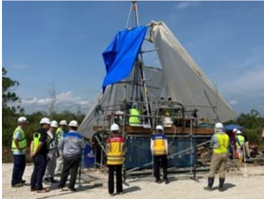
General View of Hybrid Drilling
