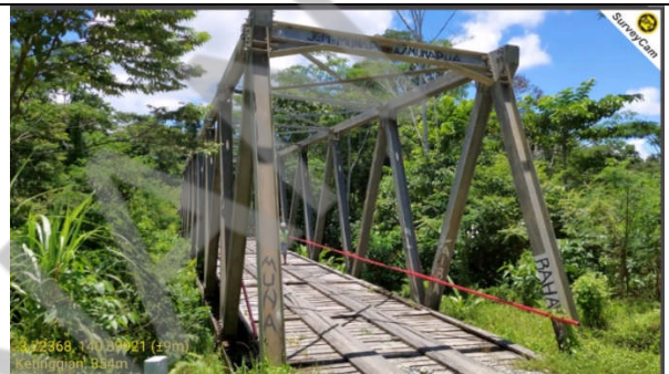
Rangka Semi Baja Semi Permanen (RBS) (BPJJN Papua Jayapura)
