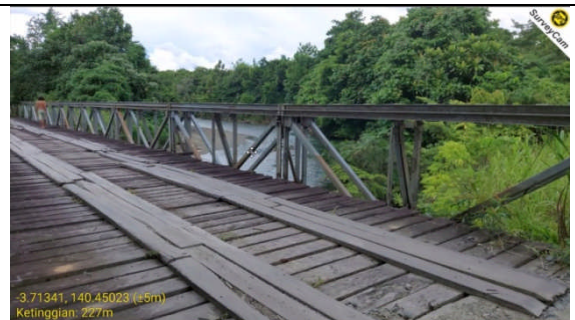
Rangka Transpanel Australia Sementara (RBS) (BPJJN Papua Jayapura)
