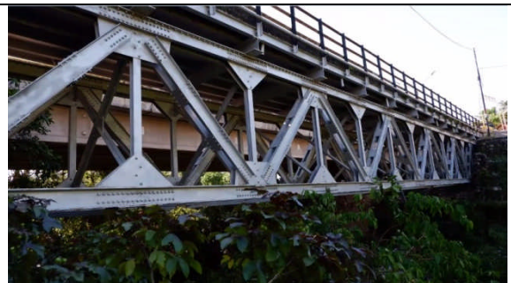
Rangka Semi Permanen (RBS) (BPJJN NTT)
