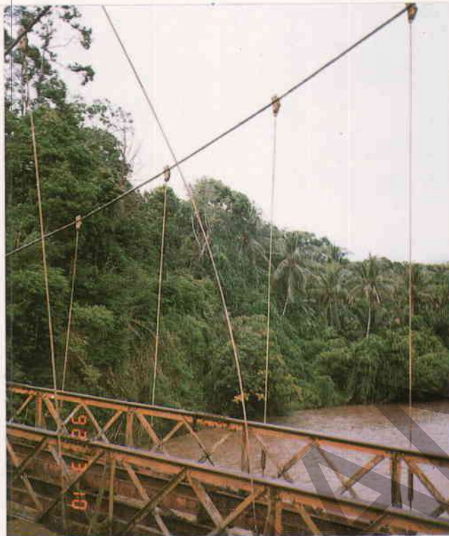
Figure A4.64 - Unsecured Hangers on Suspension Bridge Emergency Action Required
