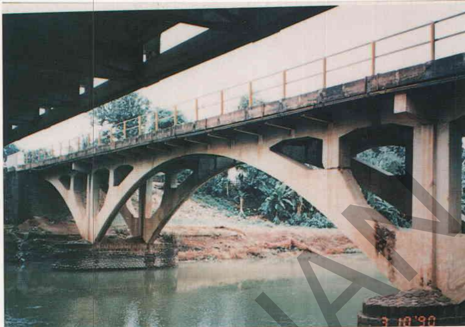
Figure A4.32 - Superstructure Type LTI Indonesian Beam Arch (under deck type)
