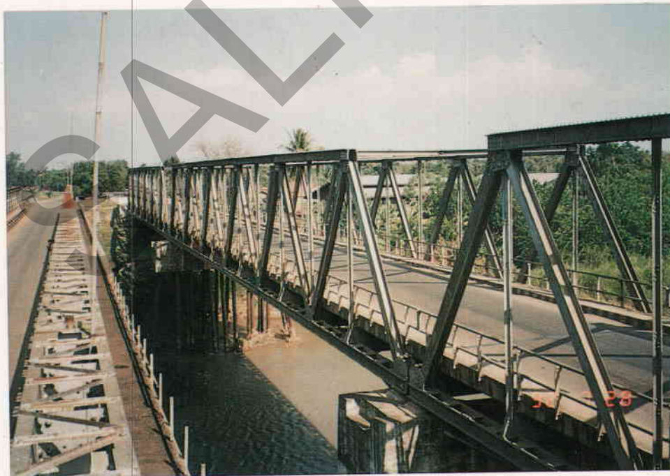
Figure A4.41 - Superstructure Type RBB New Dutch Steel Truss (Long Spans with Verticals)
