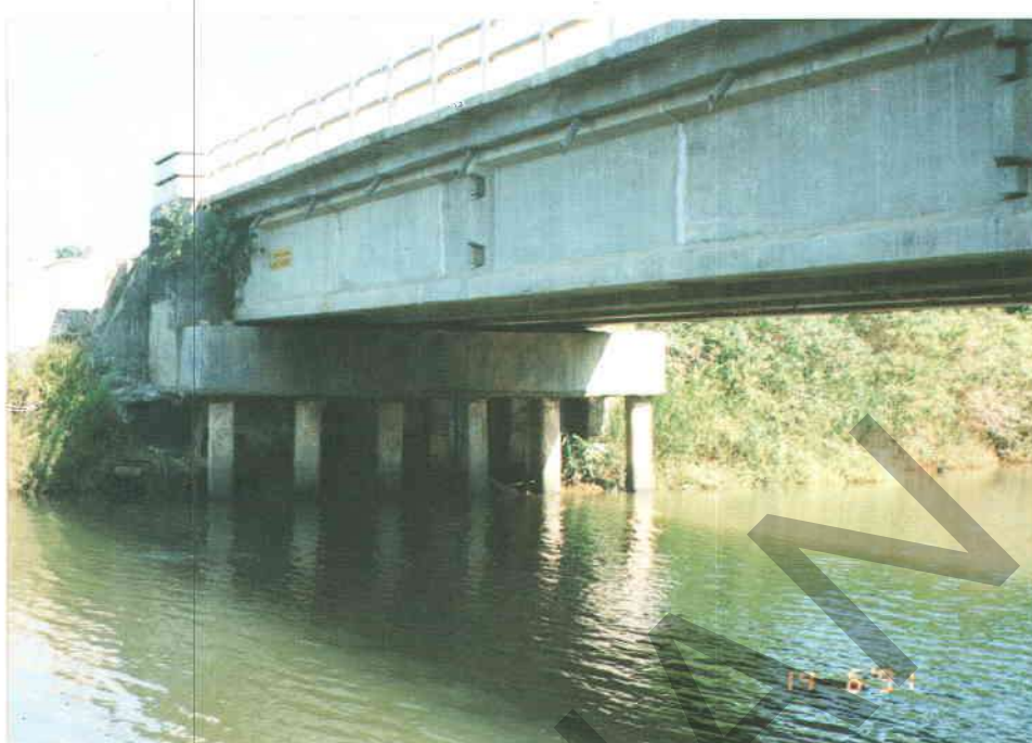
Figure A4.5 - Foundation Type T Driven Pile
