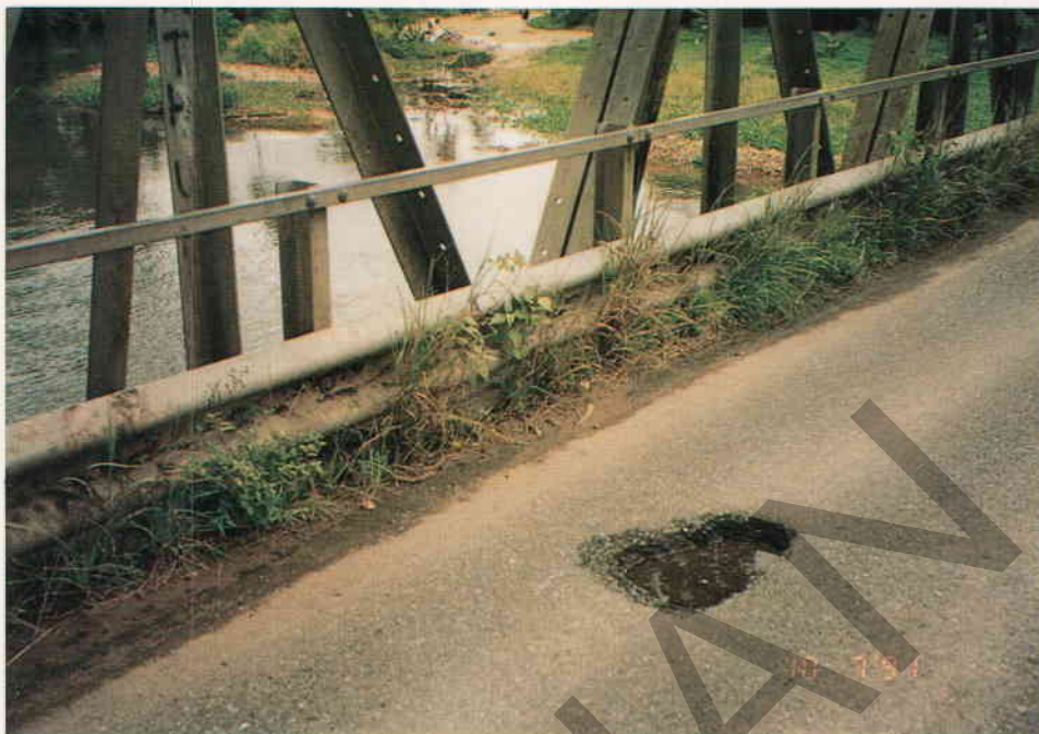
Figure A4.76 - Pot Hole in Deck and Dirt and Vegetation along Kerb needs minor repairs and cleaning
