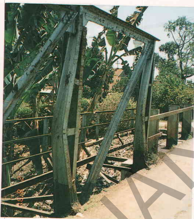
Figure A4.60 - Damaged Truss Vertical Strengthened
