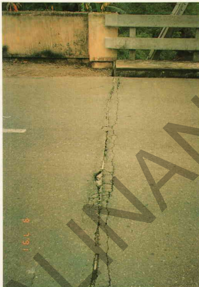
Figure A4.104 - Cracked Asphalt at Expansion Joints both Abutments
