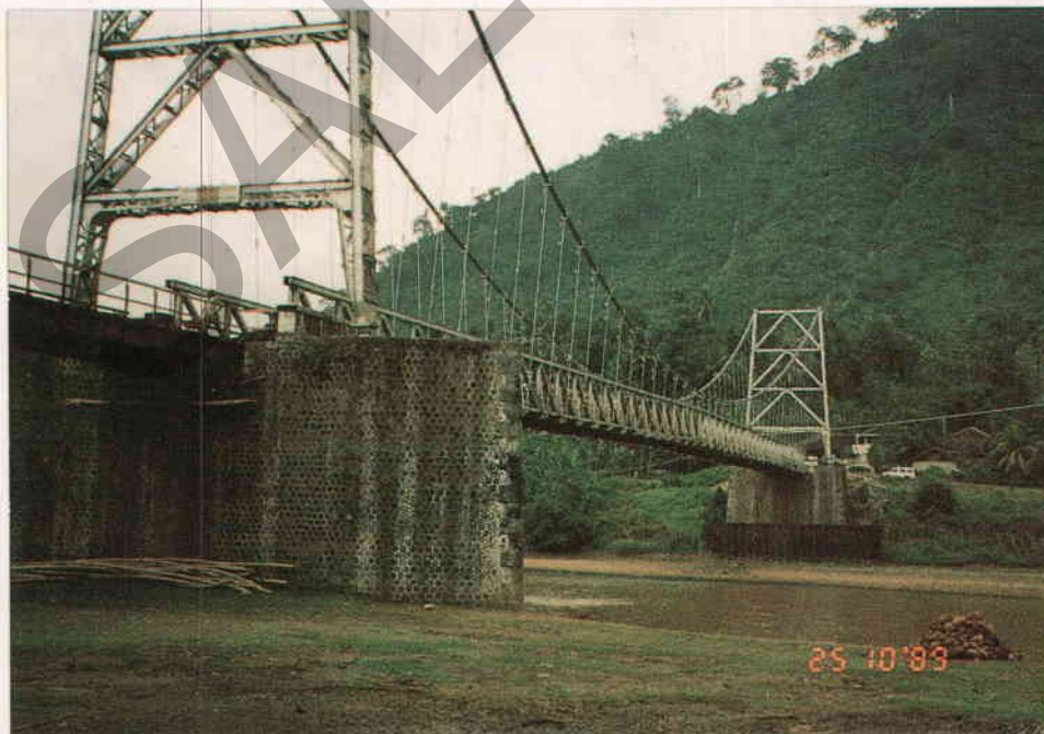
Figure A4.22 - Superstructure Type TBI Suspension Bridge
