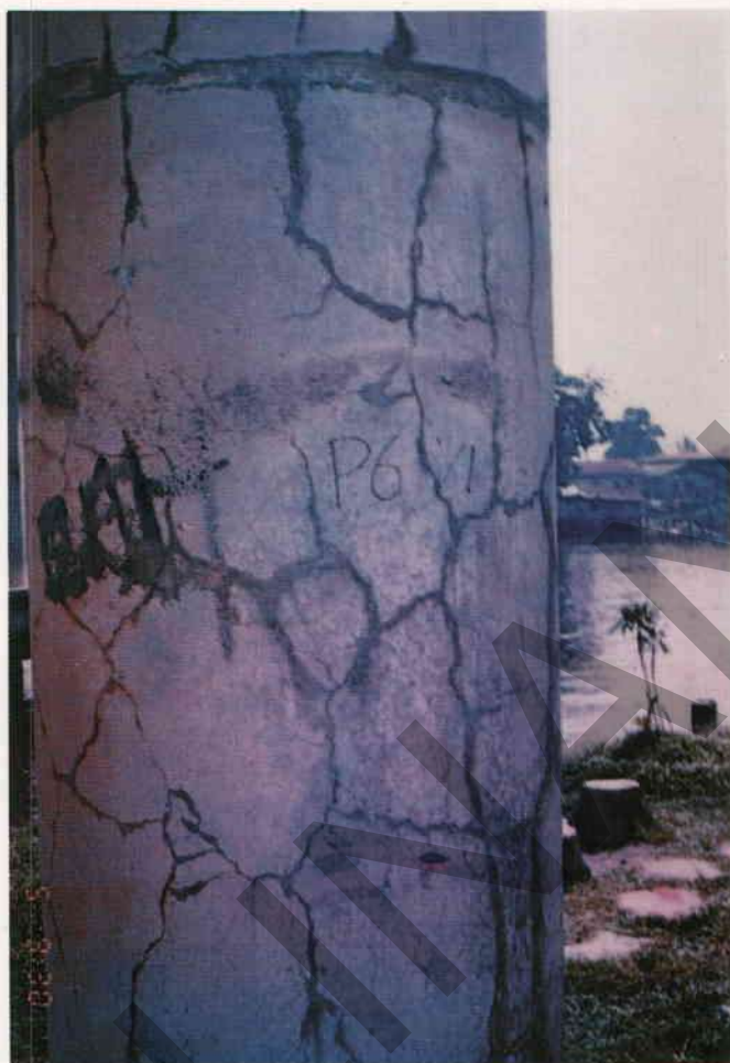
Figure A4.87 - All Columns in Pier 6 Extensively Cracked
