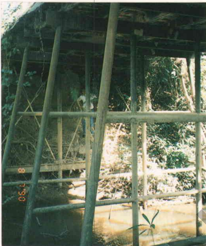
Figure A4.7 - Foundation Type TU Screw Pile
