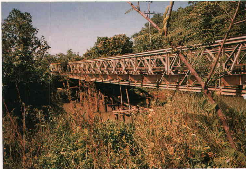
Figure A4.38 - Superstructure Type RBW/SBW Bailey Type Steel Truss Bridge (Acrow Type)
