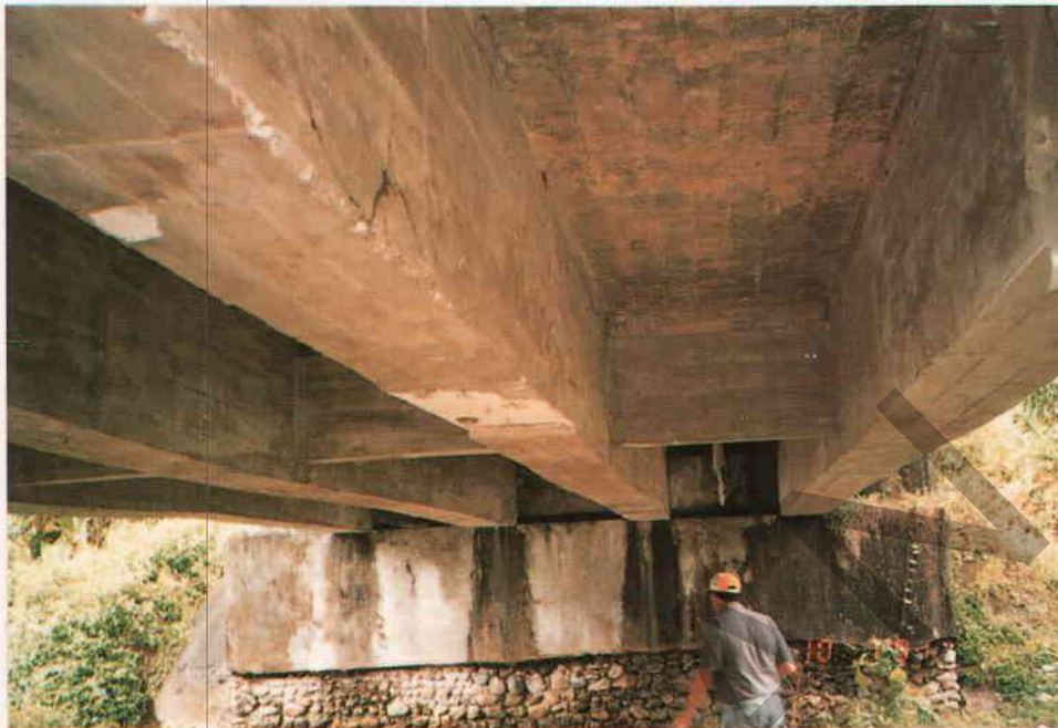
Figure A4.29 - Superstructure Type GTI Indonesian Concrete Girder (Girder Cast on Site)
