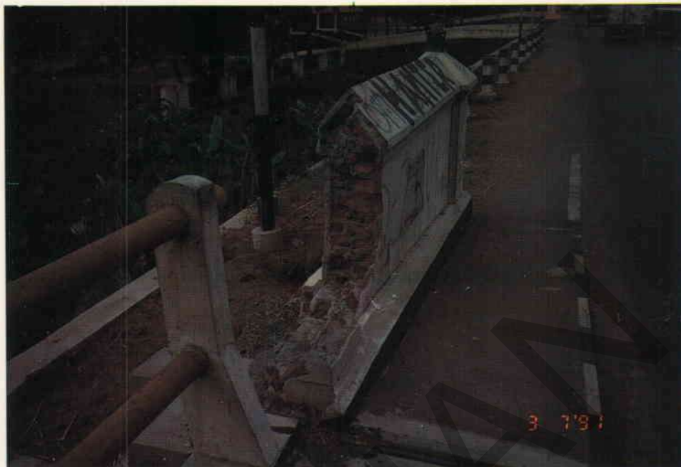
Figure A4.105 - Broken Parapet at Abutment 2
