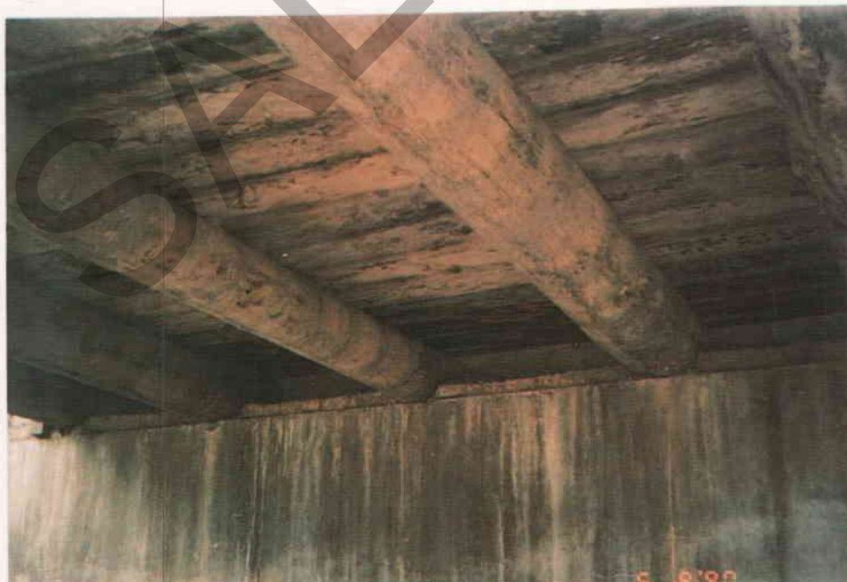
Figure A4.30 - Superstructure Type GKI Indonesian Concrete Girder
