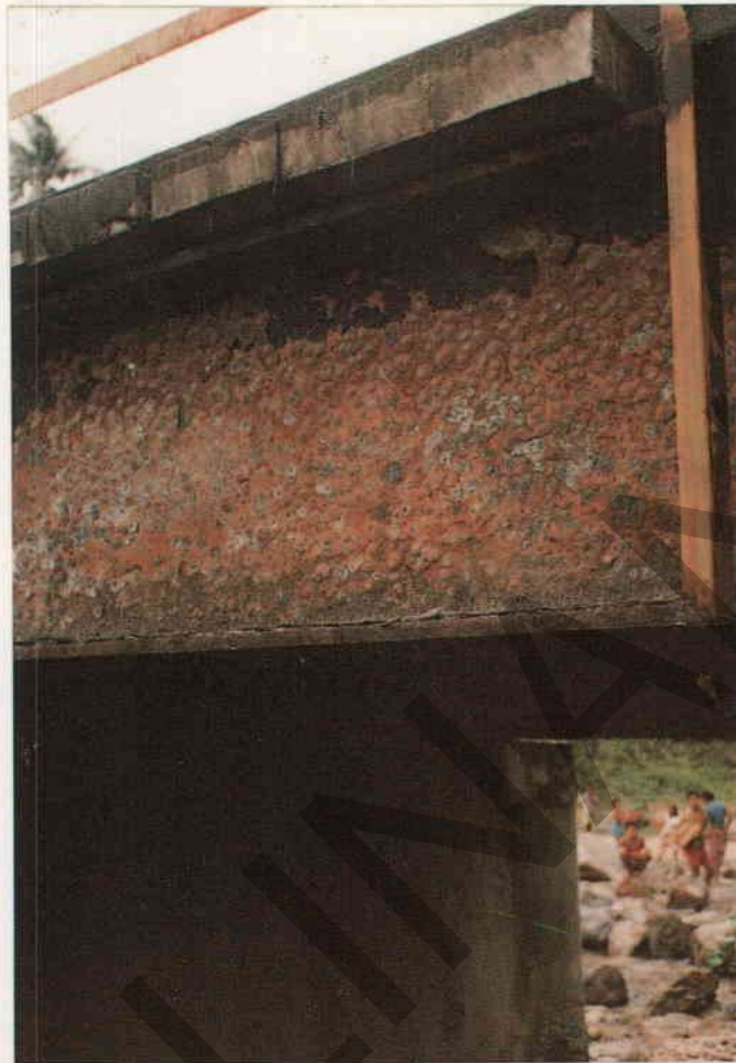
Figure A4.94 - Surface Protection Lost and Minor Corrosion of Steel on the Entire Girder System
