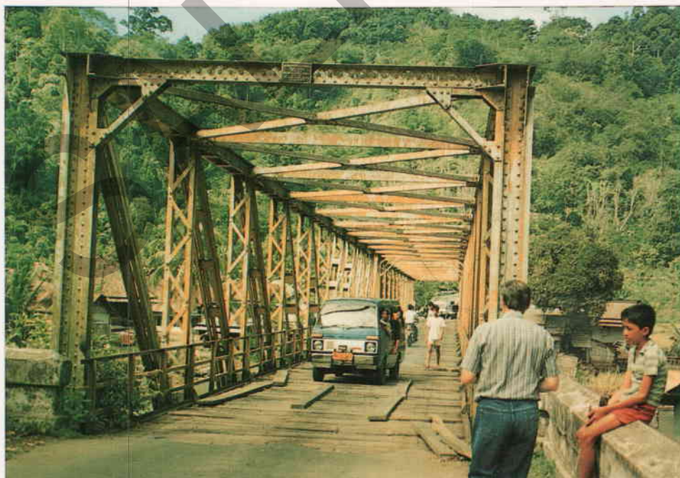
Figure A4.43 - Superstructure Type RBD Old Dutch Truss (Short Spans with no Verticals)
