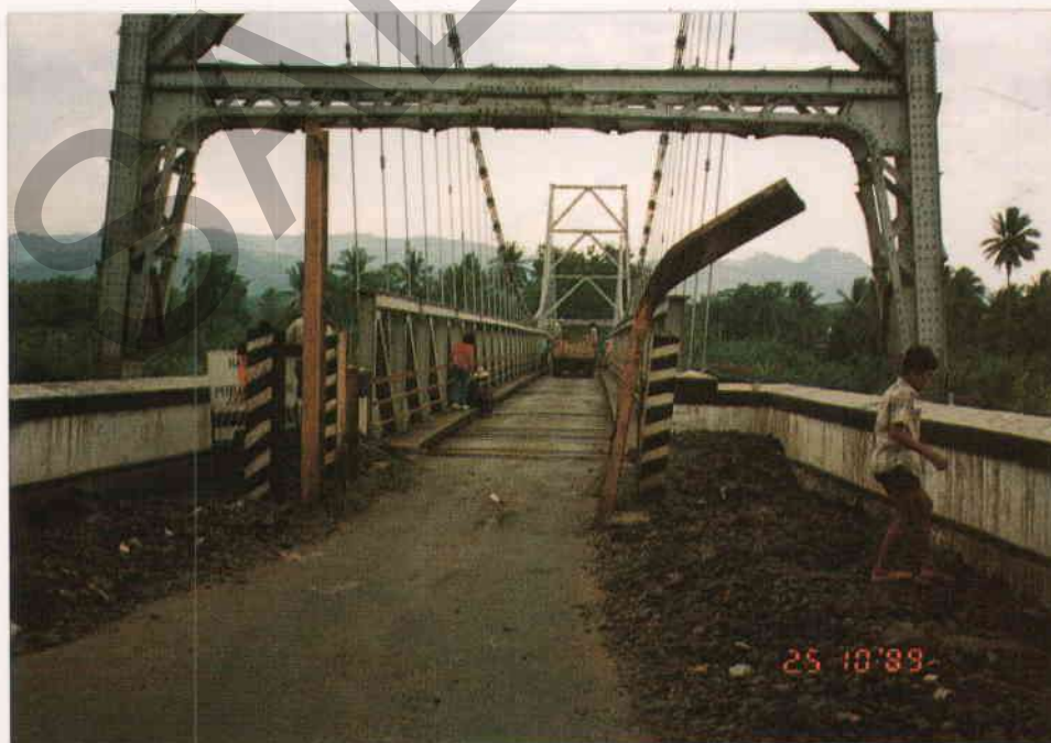
Figure A4.81 - Width Gauge Damaged by Impact
