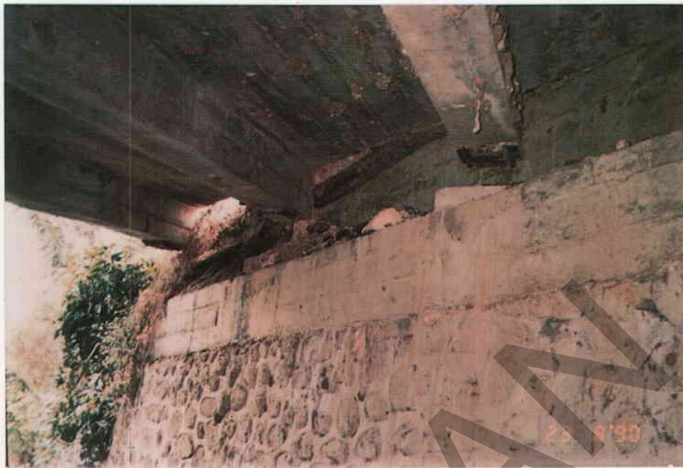
Figure A4.83 - Scouring of Foundation causing abutment to settle Deck is unsupported at both abutments
