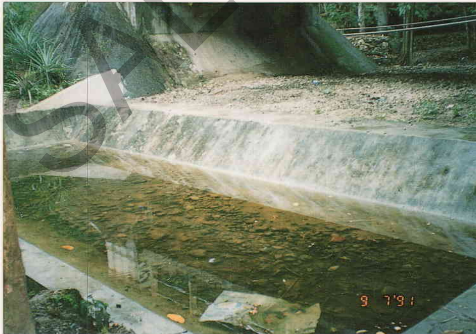
Figure A4.53 - Solution - Bottom Controller Constructed and Stream Bed Returns to Original Bed Level
