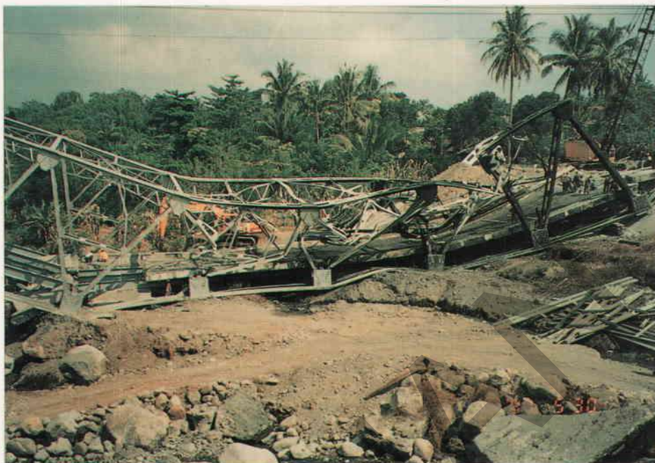
Figure A4.91 - Bridge collapsed due to fire
