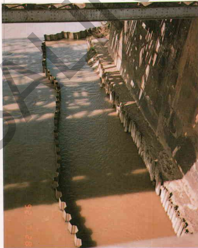
Figure A4.65 - Sheet Piles Constructed to Prevent Scouring of Abutment
