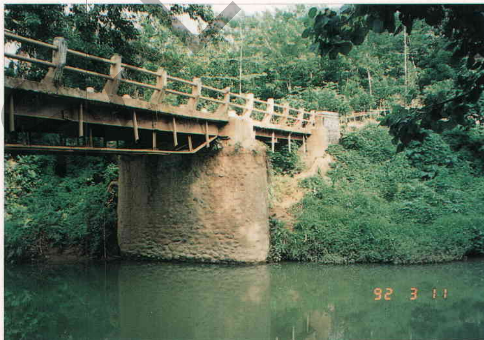
Figure A4.13 - Pier Type P Solid Wall
