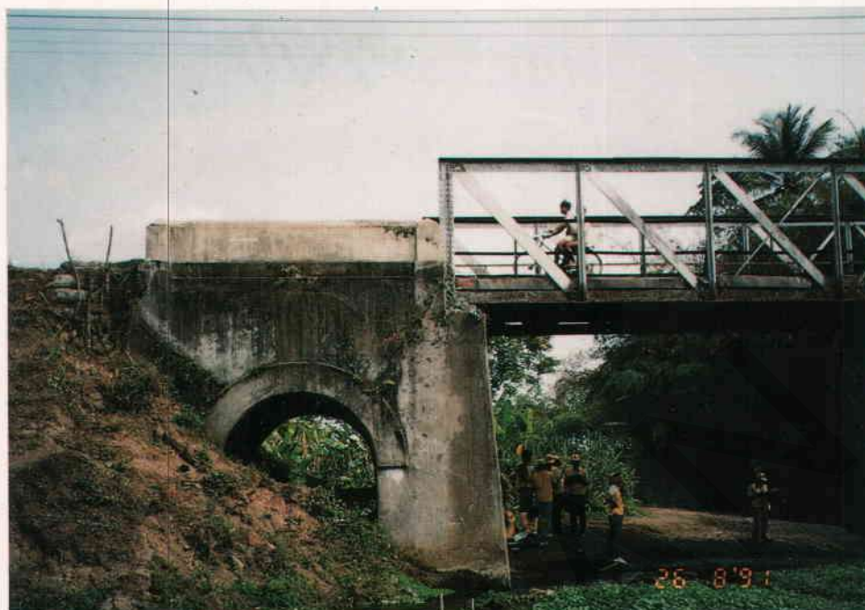
Figure A4.11 - Abutment Type K Special Abutment
