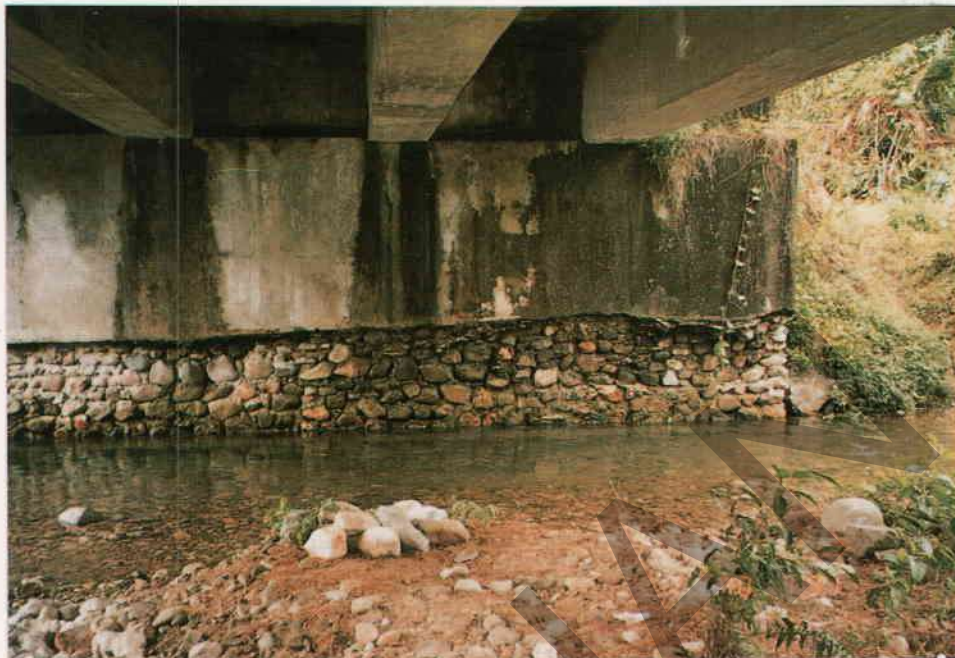
Figure A4.82 - General Degrading of Stream Bed
