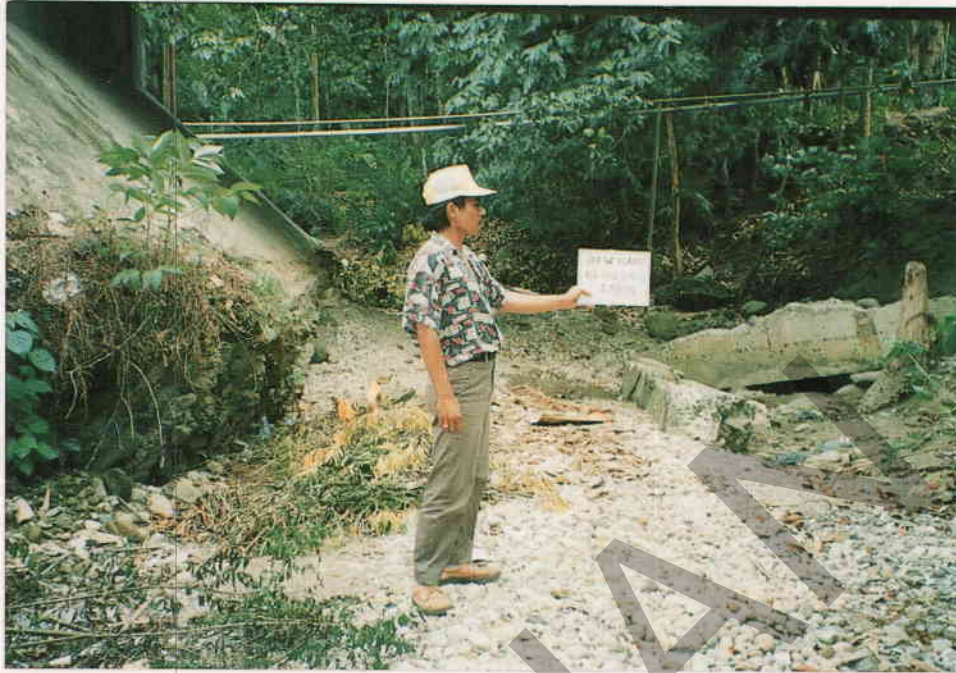
Figure A4.52 - Obstruction, Scour and Stream Degradation
