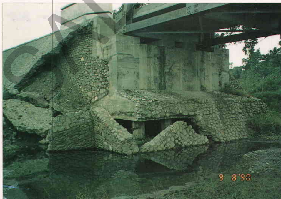
Figure A4.10 - Abutment Type B Retaining Wall
