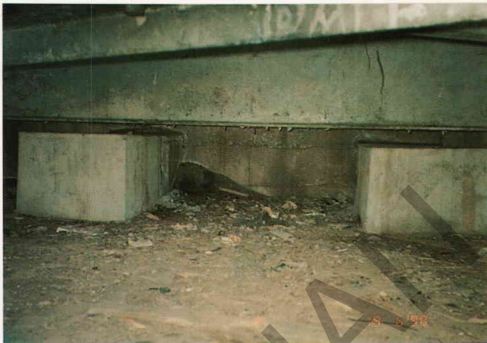
Figure A4.88 - Missing Earthquake Restraint at Abutment 2
