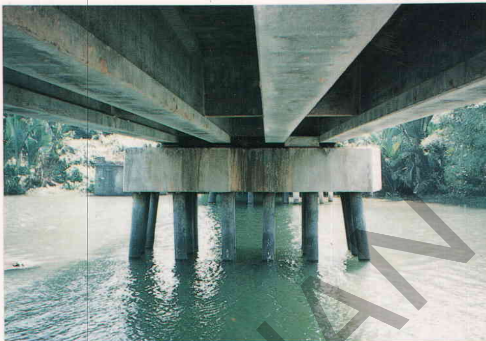
Figure A4.12 - Pier Type C Pile Cap
