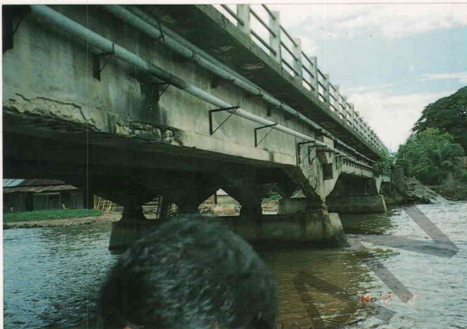
Figure A4.92 - Concrete girder system all in poor condition due to very poor quality concrete
