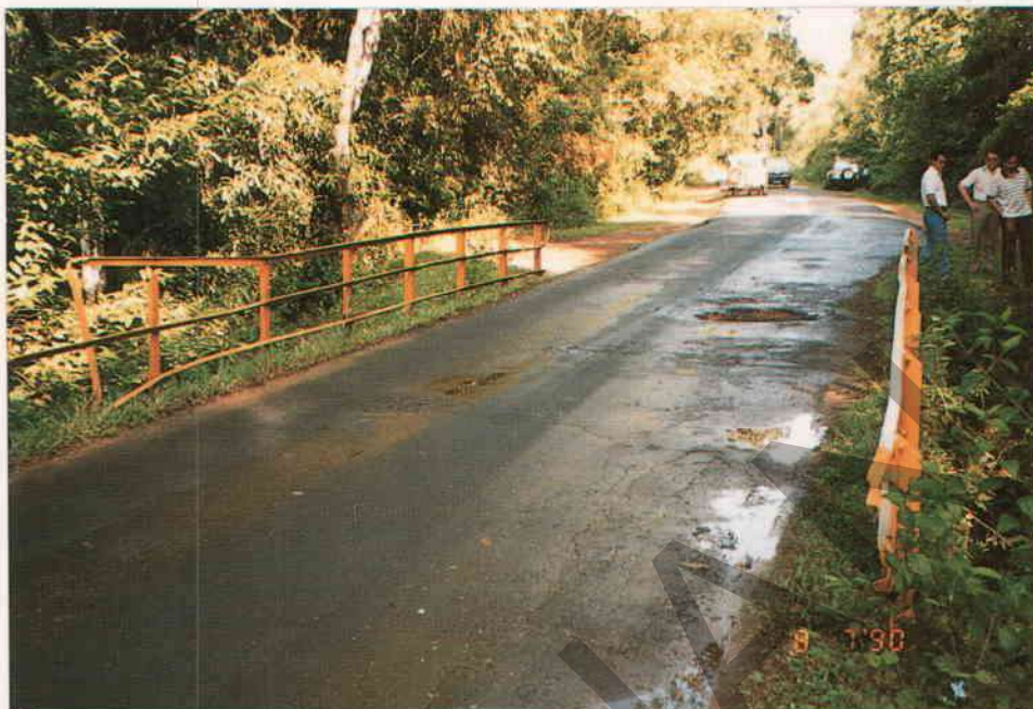
Figure A4.74 - Potholed Deck needs minor repairs
