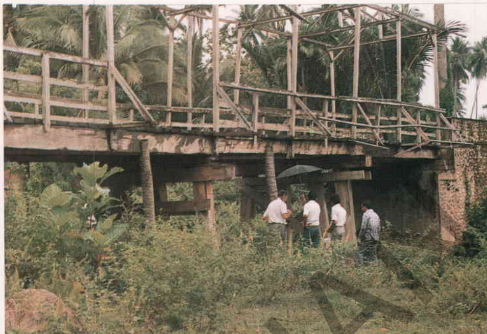
Figure A4.62 - Temporary Props under Weak Timber Girder
