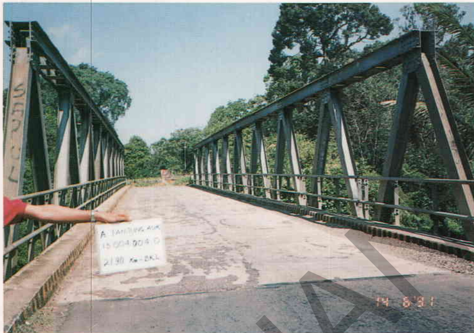
Figure A4.42 - Superstructure Type RBB New Dutch Steel Truss (Short Spans with no Verticals)
