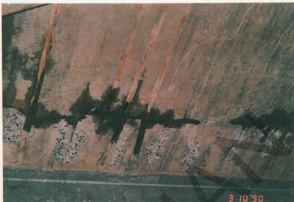
Figure A4.98 - Extensively Cracked Deck
