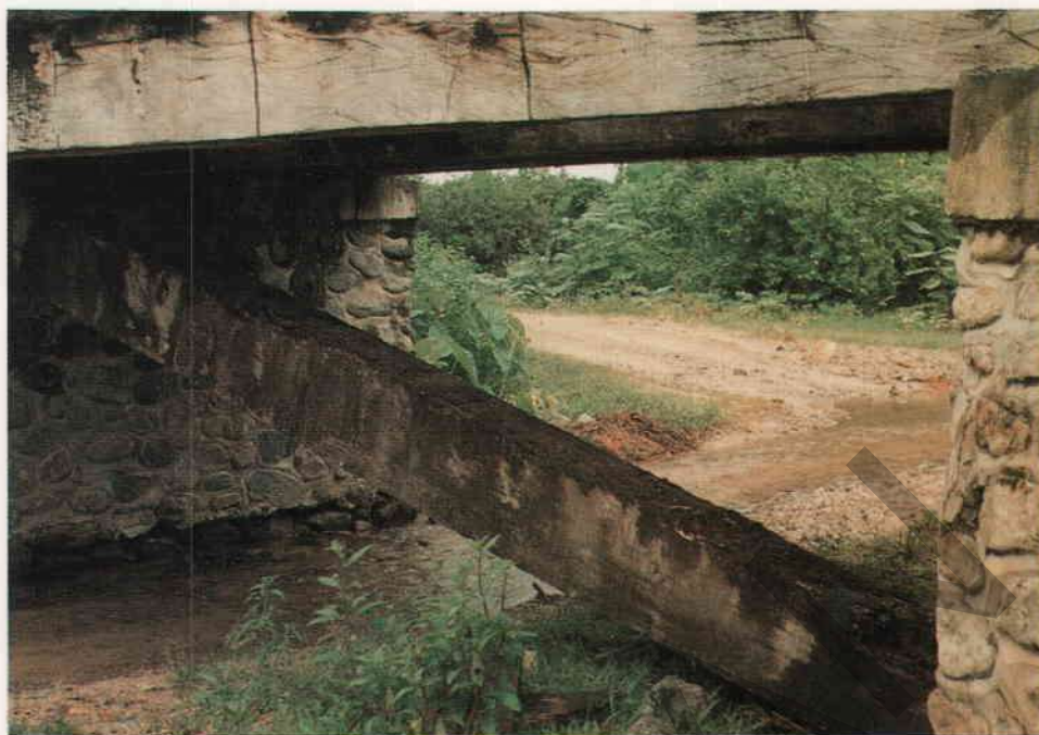
Figure A4.95 - Collapsed Girder
