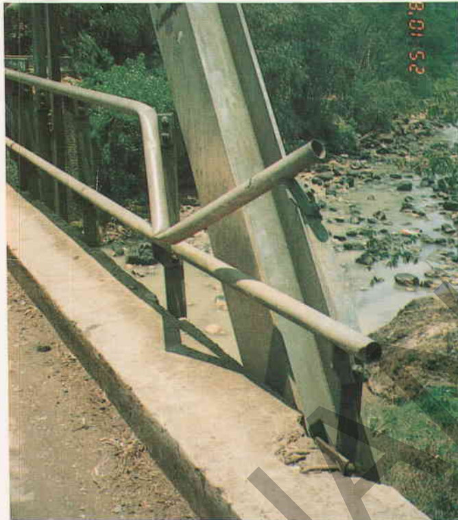
Figure A4.78 - Minor Repairs to Handrails Required
