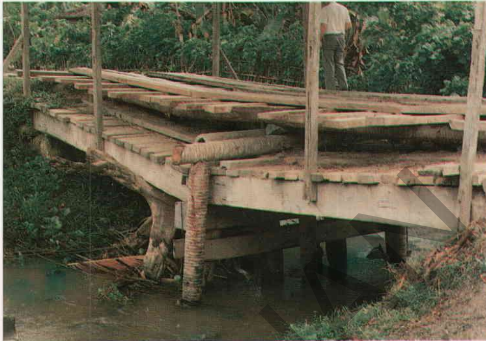
Figure A4.85 - Foundation Settlement at Pier
