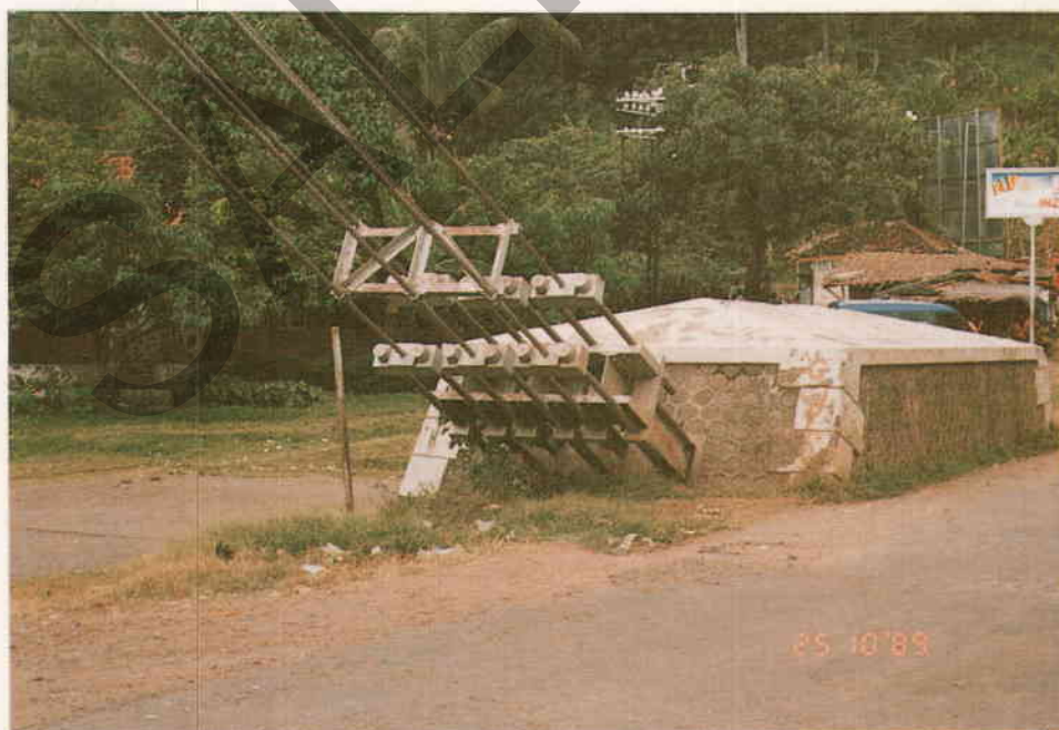
Figure A4.69 - Example of Good Routine Maintenance Keeping the Anchor Area at a Suspension Bridge Clean
