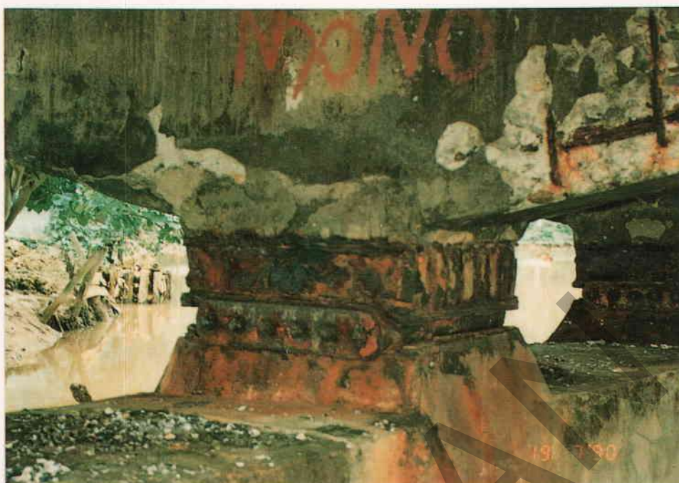
Figure A4.103 - All Bearings Siezed
