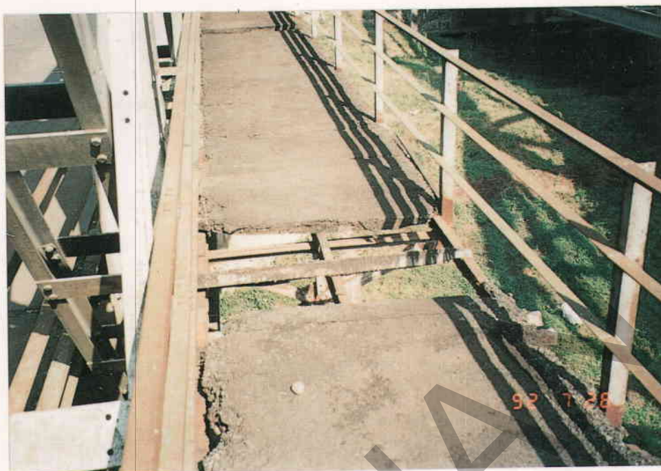
Figure A4.50 - Dangerous Walkway Emergency Action Required
