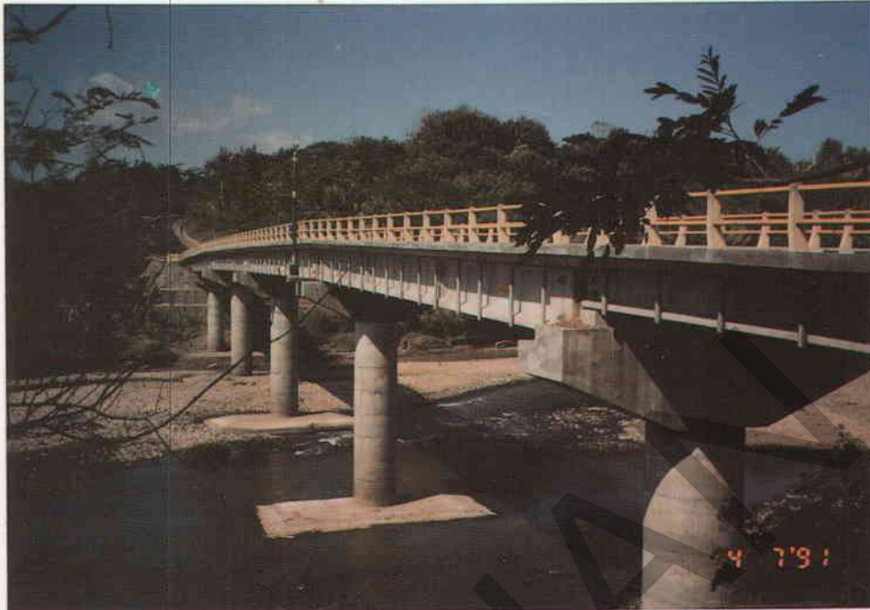
Figure A4.14 - Pier Type S Single Column
