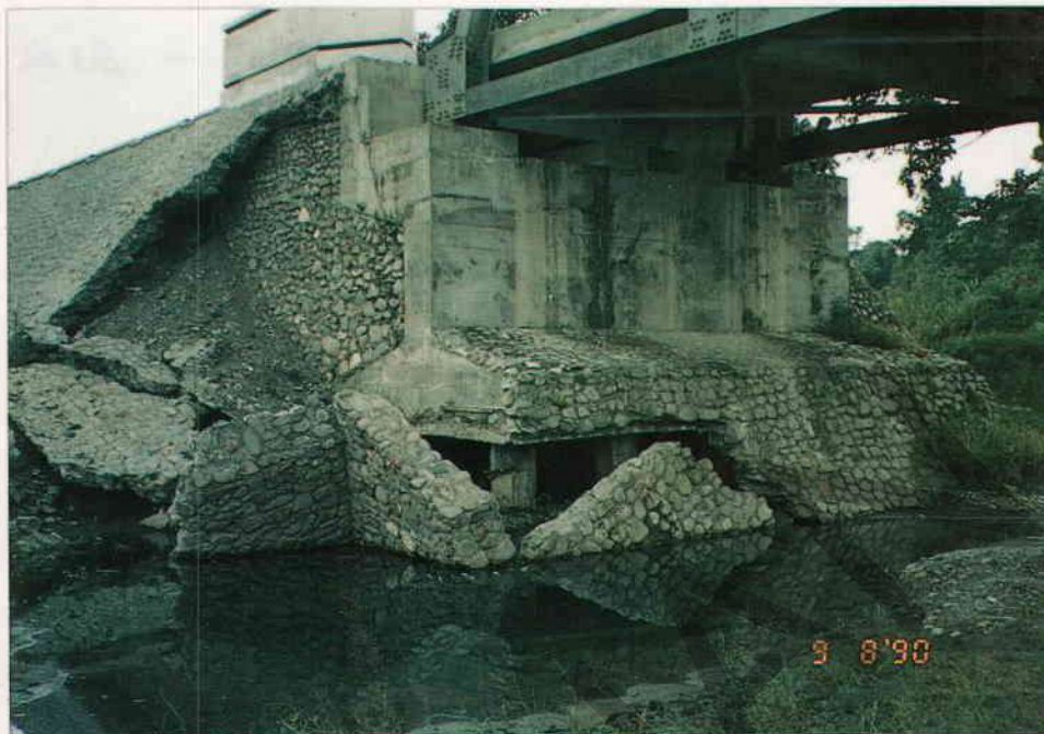
Figure A4.84 - Scour at Abutment 1
