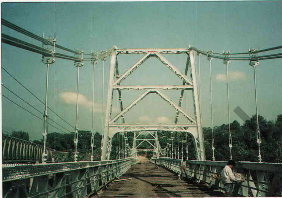
Figure A4.21 - Superstructure Type TBI Suspension Bridge
