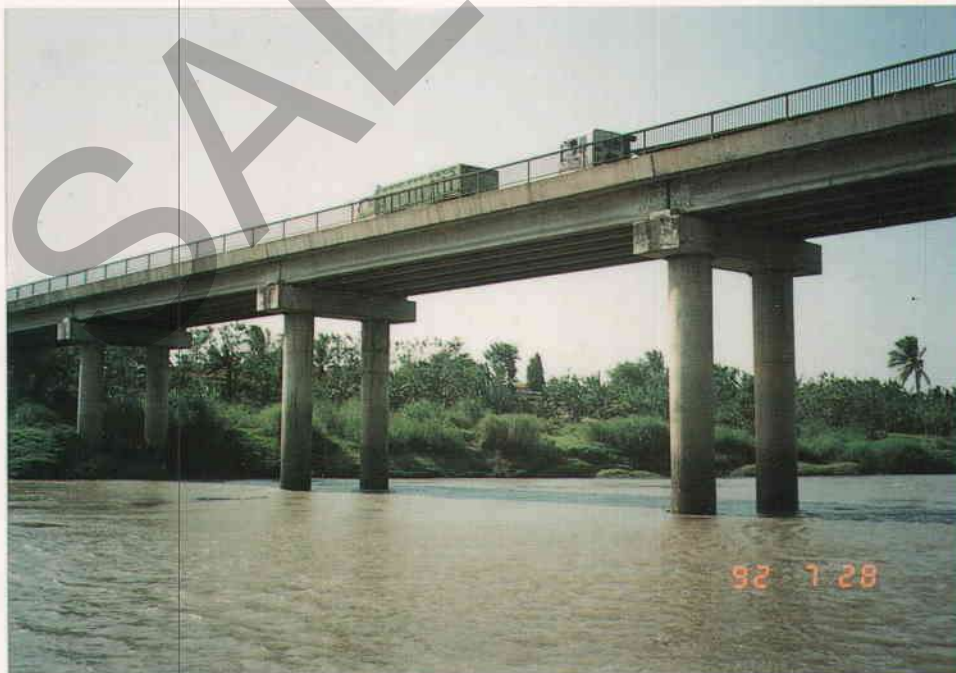
Figure A4.15 - Pier Type D Two Column
