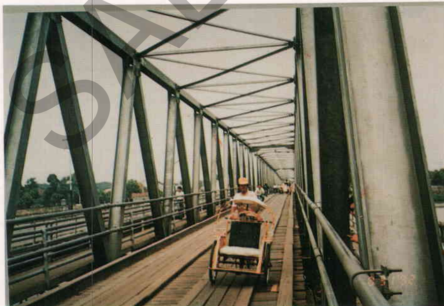
Figure A4.39 - Superstructure Type RBP Australian Steel Truss (Semi Permanent)
