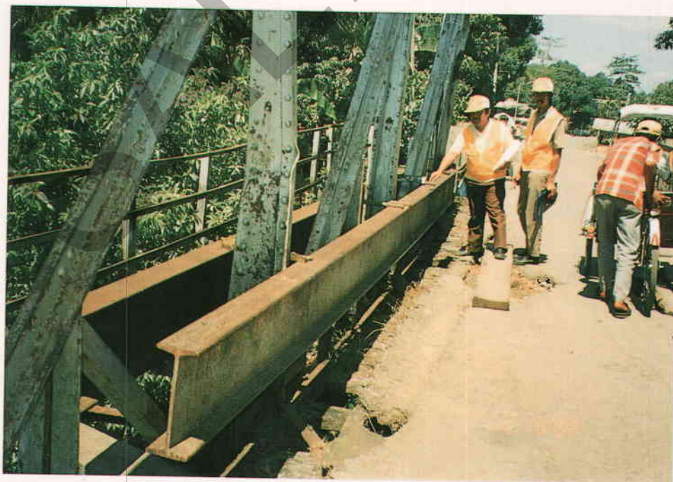
Figure A4.61 - Extra Girder Used to Redistribute Load Across Damaged Truss Section
