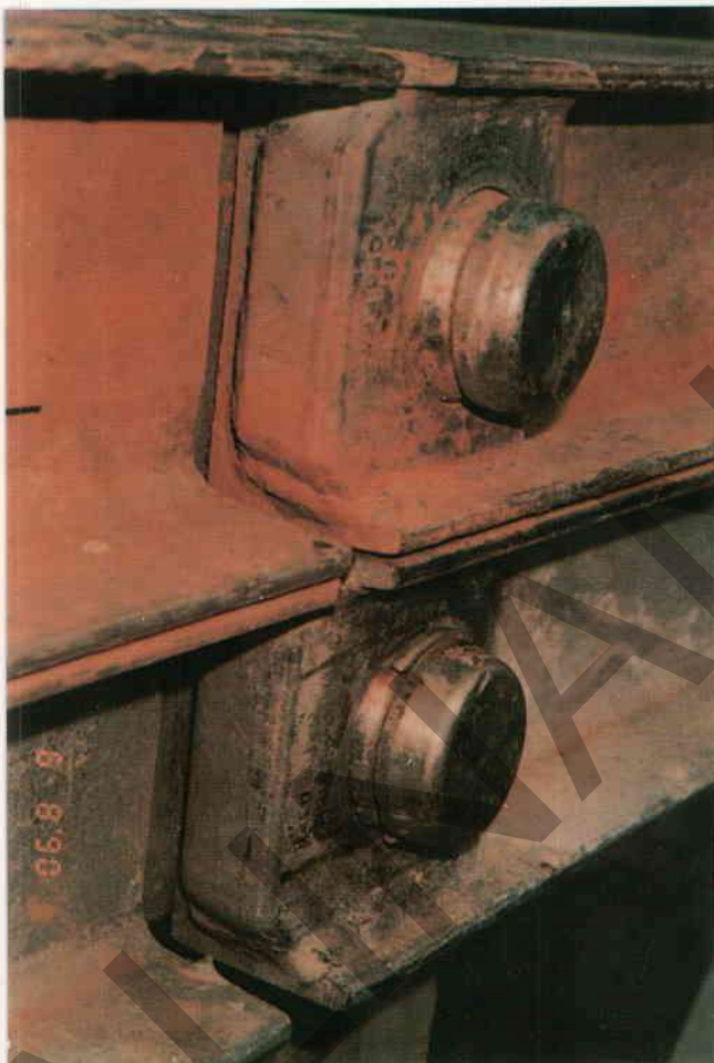
Figure A4.89 - Bridge Circlip Missing at 5th Panel on Chord on Left Side of Bridge
