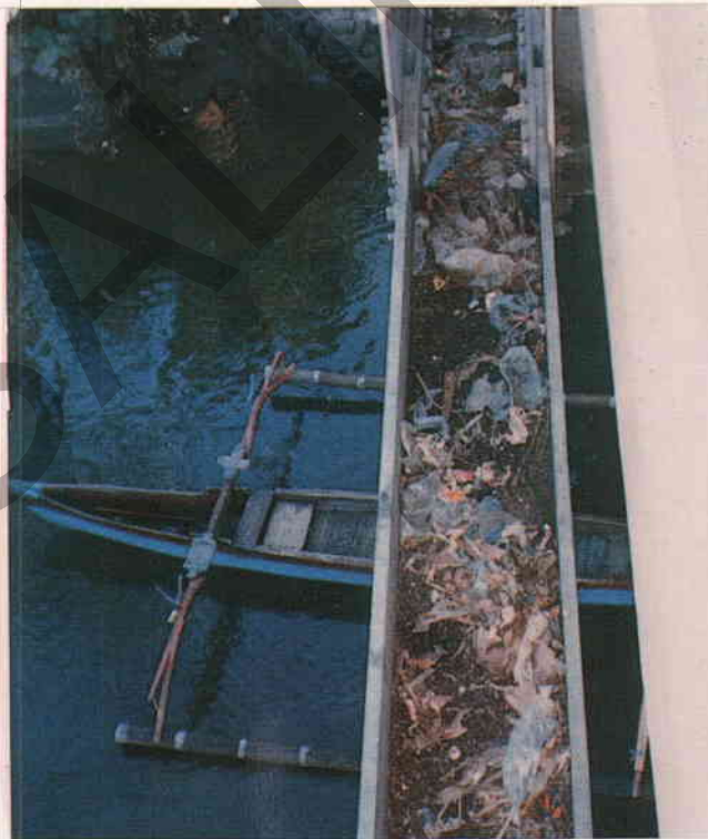
Figure A4.67 - Rubbish in Bottom Chord of Truss can accelerate corrosion Routine Maintenance Required
