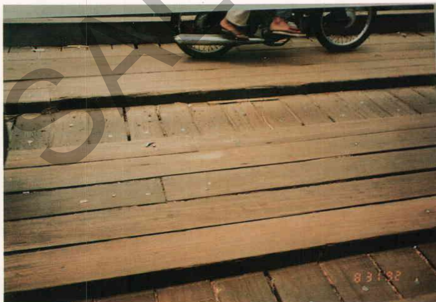
Figure A4.75 - Example of Good Routine Maintenance with Well Maintained Timber Deck Planks
