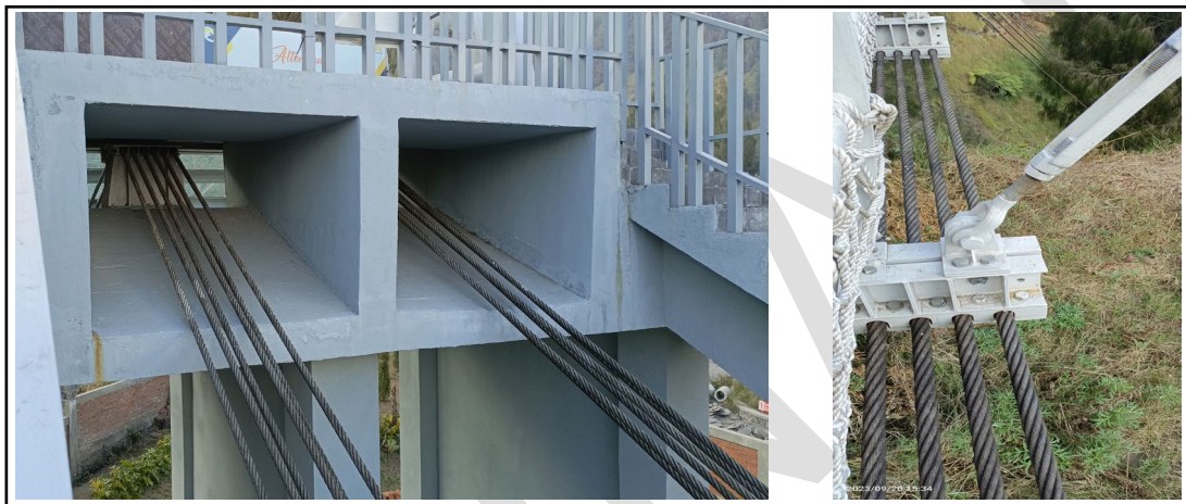
Gambar 20 - Sistem kabel suspended
