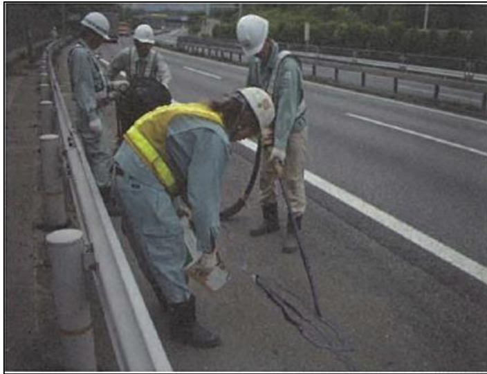
Gambar 51 – Injeksi sealant
