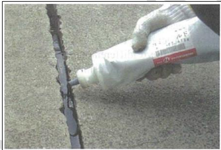
Gambar 52 – Injeksi sealant
