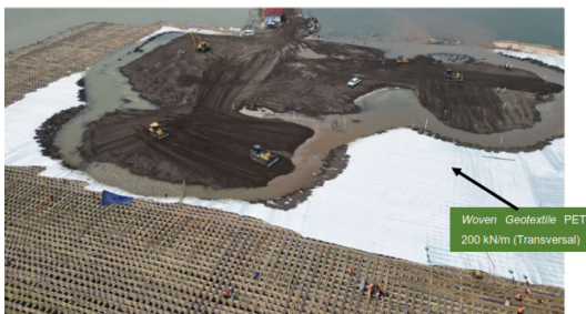
Gambar 13. Penimbunan pasir di atas geotekstil 200 kN/m (transversal) (Sumber: Work Method Statement , Satker PJT Semarang-Demak, 2023)
