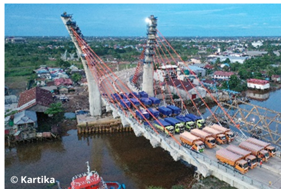
Gambar 1. Loading Test Jembatan Sei Alalak (Sore Hari)
