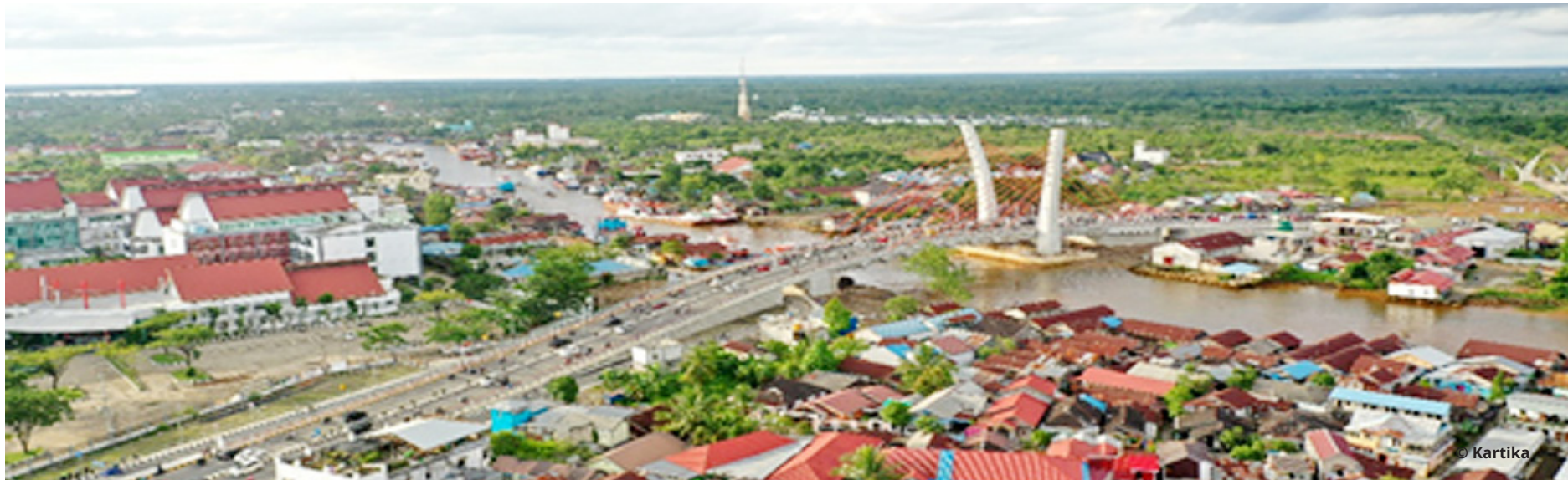
Open Traffic Jembatan Sei Alalak
