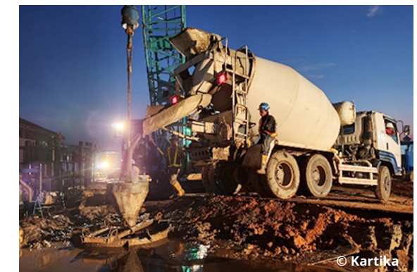
Gambar 6. Pengecoran Bored Pile
