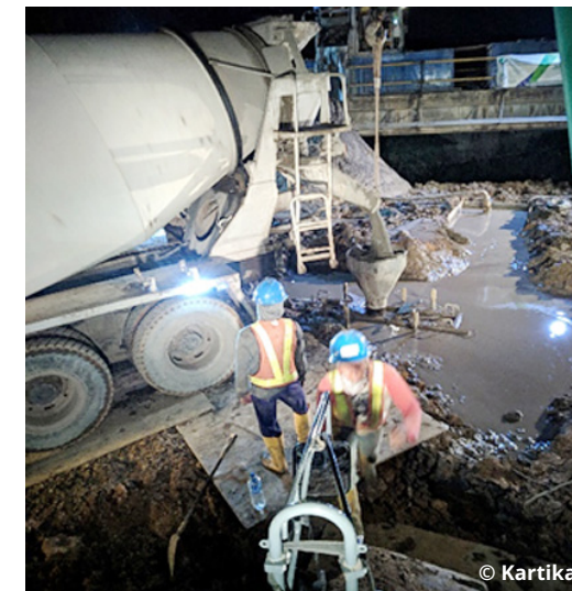
Gambar 5. Pengecoran Bored Pile
