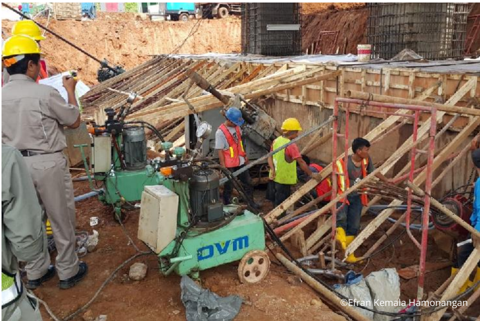
Gambar 10. Pekerjaan Ground Anchore
