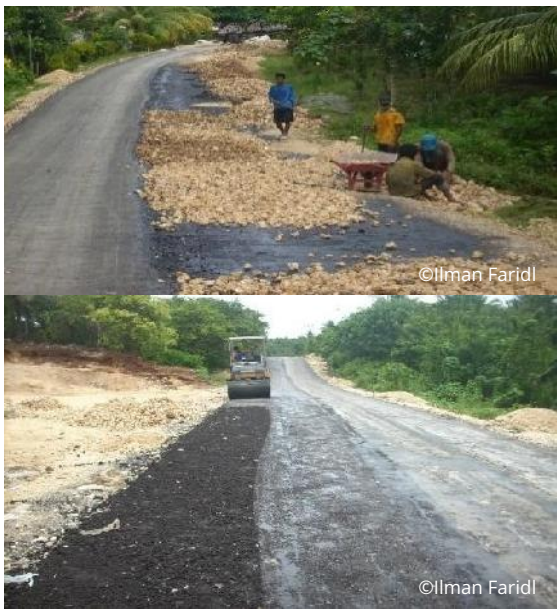
Gambar 12. Lapis Penetrasi Macadam Asbuton, LPMA, (Buton 2010)
