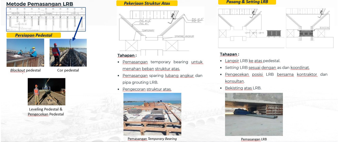
Gambar 4. Metode Pemasangan Lead Rubber Bearing (LRB)
