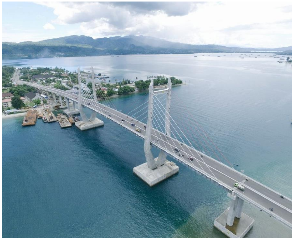
Fig. 1 Jembatan Merah Putih Cable-stayed bridge (Kementerian PUPR 2016)
