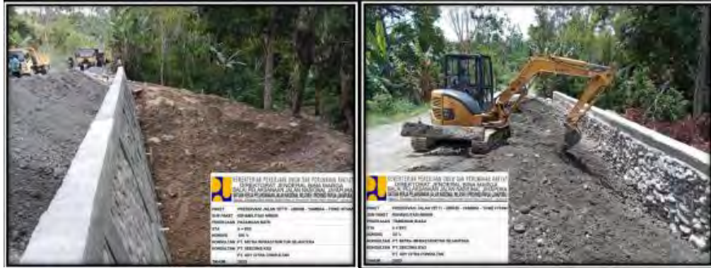
Gambar 4.18 Preservasi Jalan Yetti-Ubrub-Yambra-Towe Hitam
