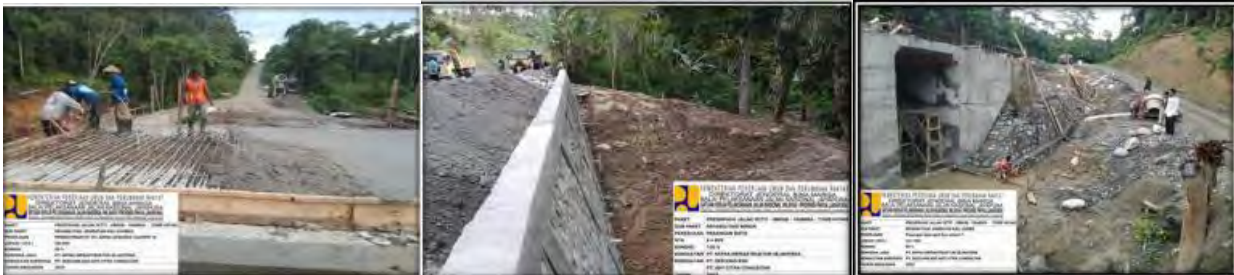
Gambar 4.23 Preservasi Jalan Yetti-Ubrub-Yambra-Towe Hitam
