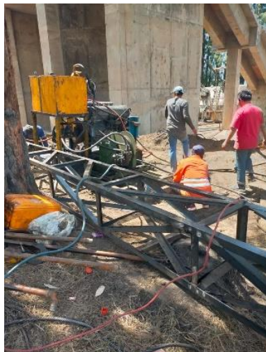
Proses Instalasi Soil Nailing
